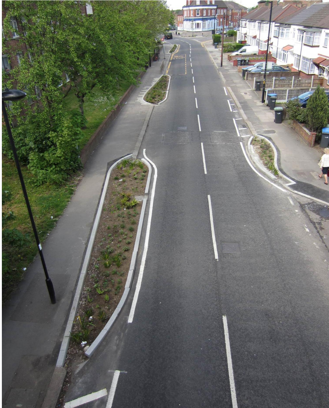
ENFIELD – Using gravel filter medium – approximately 30% void
