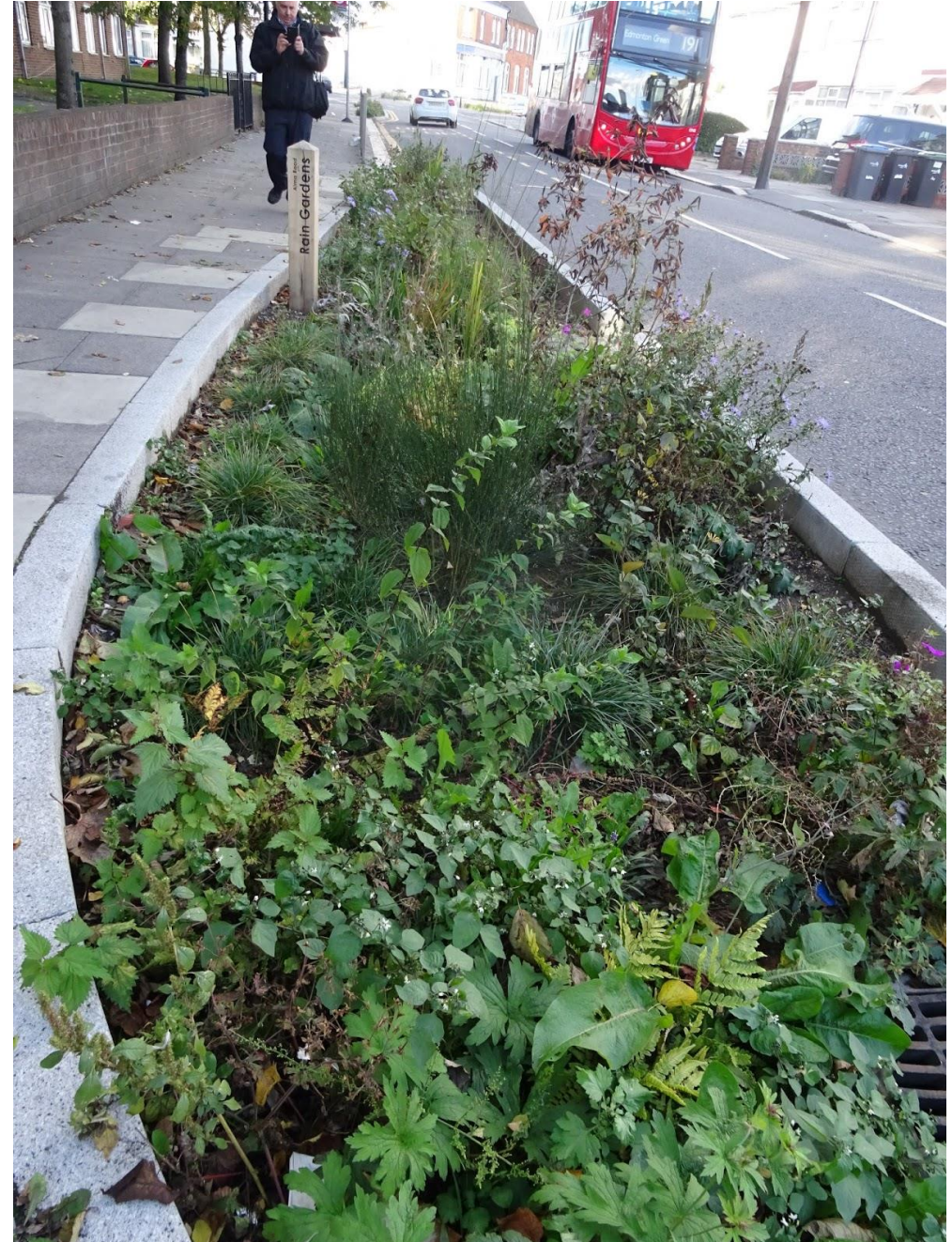
ENFIELD – Using gravel filter medium – approximately 30% void
